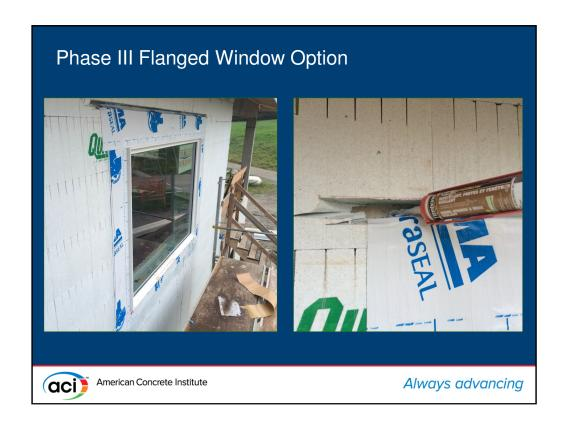
For the flanged-window module, the head-flashing was sealed directly to the concrete, which was exposed in the reglet cut above the opening.
