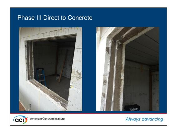
These are "post-mortem" photos of the most successful example, where the window was sealed directly to the concrete.
