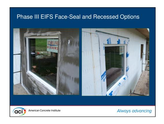
These photos show the EIFS example (left) and a treated-wood buckout (right) flashed with self-adhered membrane.
