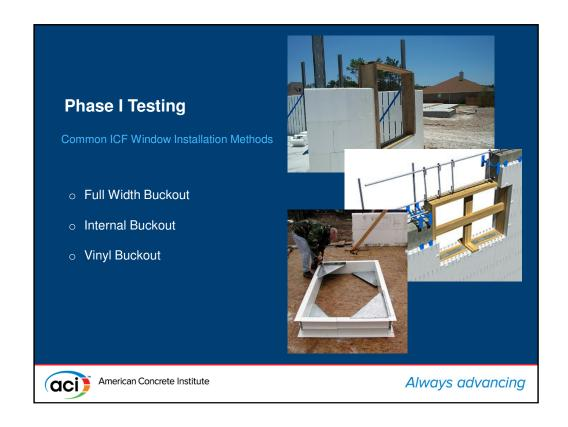
The 3 key techniques found in the industry included full-width lumber buckouts (called "exterior" bucks) that spanned from one side of the ICF assembly to the other.
